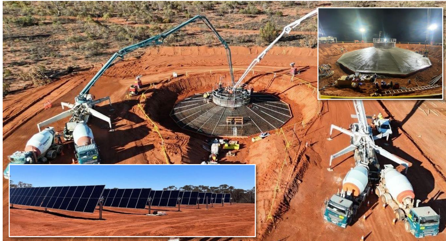
Tropicana Construction Progress
